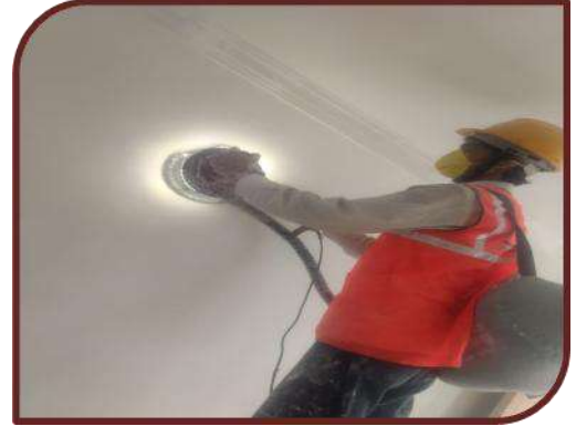
Wall leveling work at site
