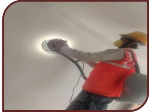
Wall leveling work at site
